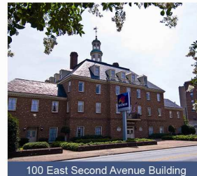
100 East Second Avenue Building
